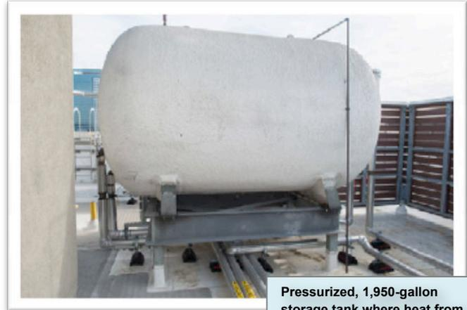
Pressurized, 1,950-gallon storage tank where heat from the solar collectors is stored, awaiting a call for hot water. When demand is low-to-moderate and the tank is hot enough, it can meet all the domestic hot water needs of the building it serves without the
