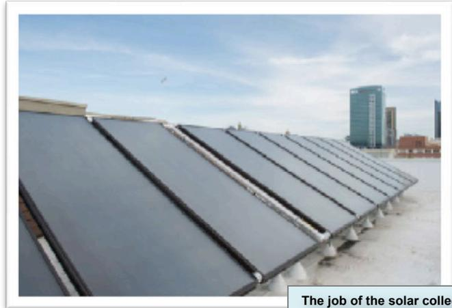
The job of the solar collectors is to boost the temperature of the incoming water supply, so that the tankless units need not work so hard to meet the set point temperature of 120°F.
