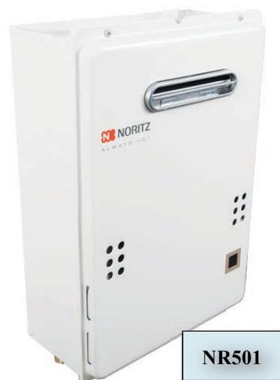
“The scale detection software and the integral display window are designed to alert homeowners and service contractors of scale buildup within the unit,” explains Noritz marketing manager Jason Fleming. “The main benefit of this early alert system is proactive leak prevention, of course. But thanks to the more durable heat exchanger, these units won’t need to be flushed as often to assure a ready and abundant supply of hot water for the household.”
