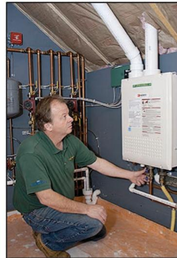
**Installer Chuck Appleby checks one of the two Noritz NRC98 condensing tankless water heaters. Condensing technology permits venting with PVC piping.**
