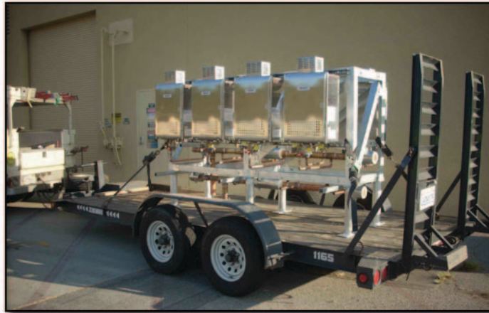
Prefabricated rack assembly of eight Noritz tankless water heaters staged on a flatbed trailer for shipment to one of the four CSUN apartment buildings in Northridge, Calif. Project manager Dan Boulais of Suttles Plumbing estimates that prefabrication cut “overall labor time in half.”
